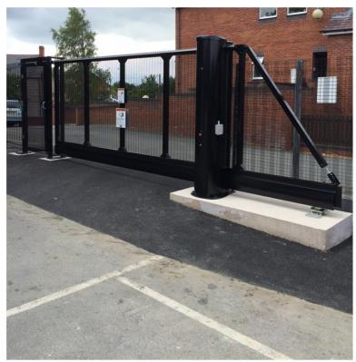
Additional safety loops can be added to increase the level of safety for vehicles if required.
