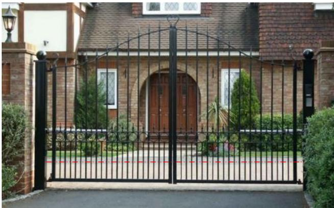
***This gate uses a combination of careful design to eliminate hinge gap hazards and drives with built in obstacle detection. The gate will stop and reverse on contact with obstacles; this is backed up by light beams across the opening.***
